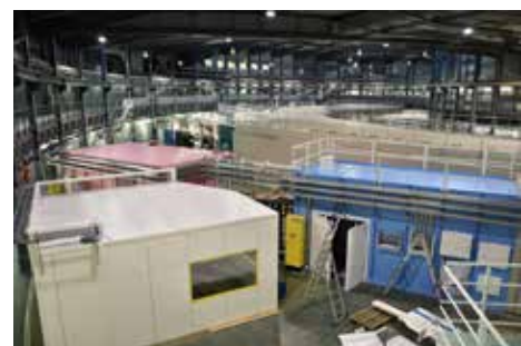
Figure 3. Optical hutch (blue), experimental hutch (pink) and control hutch (white) of XAIRA beamline.
